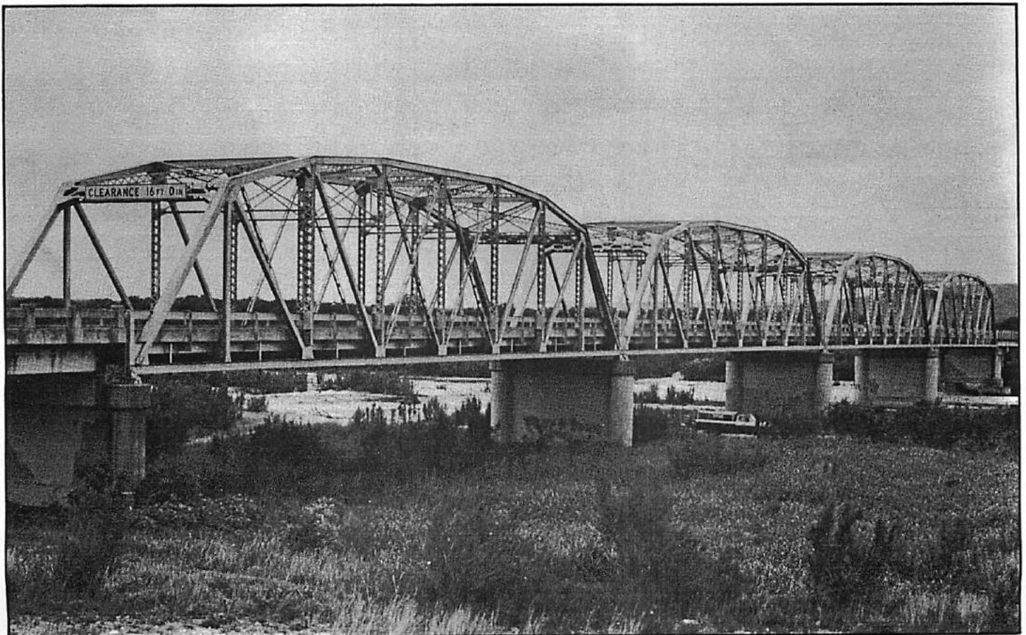
Steel truss bridge over the Nueces River, Uvalde County.
